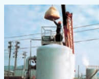
Filter media replacement work
