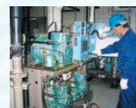
Chemical cleaning work for refrigeration air conditioners
