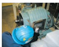
Blower inspection and maintenance
